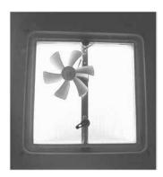
The roof vents are operated from inside and have built-in screens. To operate, turn the crank in the center of the vent clockwise to open and adjust. The bath vent may be equipped with a 12-volt exhaust fan. The switch to control the fan is located on the vent. These vents may be left slightly open while traveling, but be careful when traveling where vertical clearance is limited. Vent lids can crack if left open too far.
