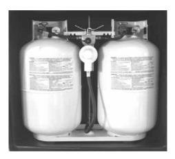
Dual propane tanks are equipped with a two-stage automatic changeover regulator, which transfers propane demand automatically to the second tank when the first tank becomes empty.
